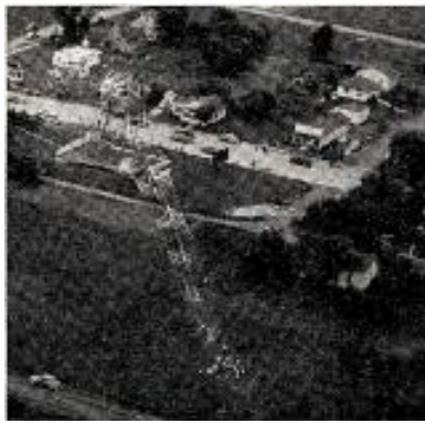
A TORNADO, which twisted through Rice Lake, Wis., June 24, destroyed the 454-foot tower of WJMC-AM-FM. Thanks largely to WJMC engineers, the station lost only 9 hours, 40 minutes of operating time.
